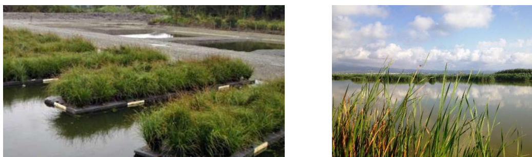
Figure 4-17: Artificial wetlands/green filters are used as purification systems to improve water quality. Typically, wetlands are constructed to provide secondary and tertiary treatment of wastewater and improve local water quality
