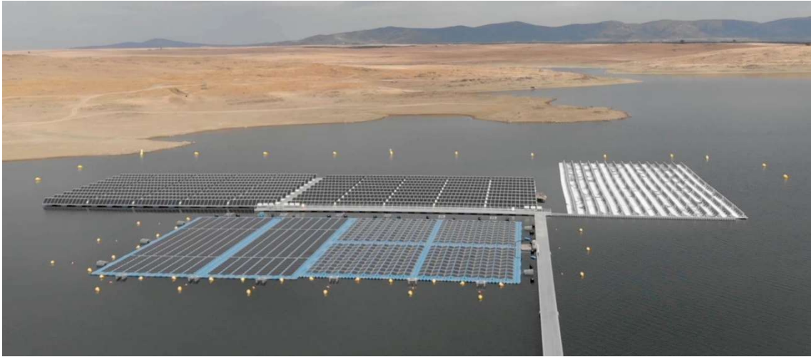
Figure 4-13: Evaporation losses in lakes and reservoirs amount to more than 350 km 3 per year. One possible solution is to cover part of the reservoir surface with solar panels, thus achieving a double function: reducing losses and energy production (Image of the floating photovoltaic plant in the Sierra Brava reservoir in Spain).
