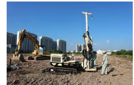
Figure .4 On-site Well Construction
