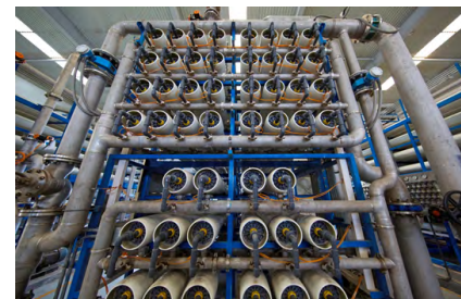
Figure .1 The Reverse Osmosis Equipment of the Sewage Treatment Plant
