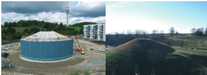
Figure 1 – Large Hot Water Storage (construction and final state) combined with Solar Thermal District Heating “Am Ackermann-bogen” in Munich, Germany
