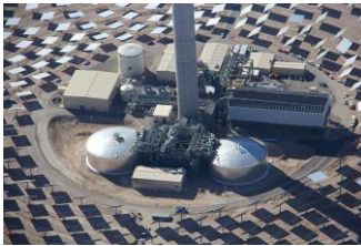
Fig. 63 and 64: CSP-plants with mirror (left) and trough (right) system and integrated storage tanks using molten salt [32], [33]
