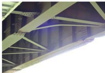
Buckling of girder
