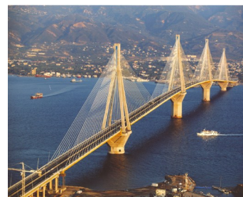
Rio - Antirrio Suspended Bridge, Greece
