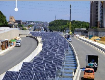
Solar power panel + bicycle path
