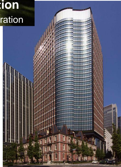
Marunouchi Park Building
