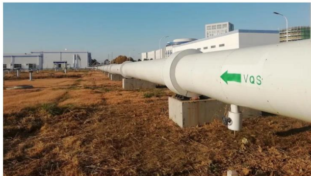
A pipeline carrying heated water from the Haiyang plant (Image: SPIQ)
