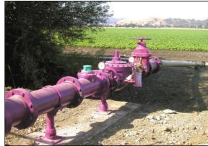
Purple lines to convey treated water
