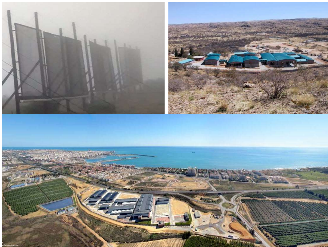
Figure 4-19: Unconventional resources are essential in areas where water scarcity has become structural or necessary to release other water resources for environmental purposes. Fog water harvesting can provide between 2 to 10 l/m 2 per day (in the image above left, fog harvesting meshes in Chile). Water reuse treatments make it possible to reuse the resource mainly for agriculture. However, in some countries, such as Namibia, it is used for water supply (in the image above right, water reuse plant in New Goreangab, Namibia). Desalination by reverse osmosis has grown exponentially over the last few decades, mainly due to the drastic reduction in energy consumption (in the image below, Torrevieja desalination plant -240,000 m 3 /day-, Spain).
