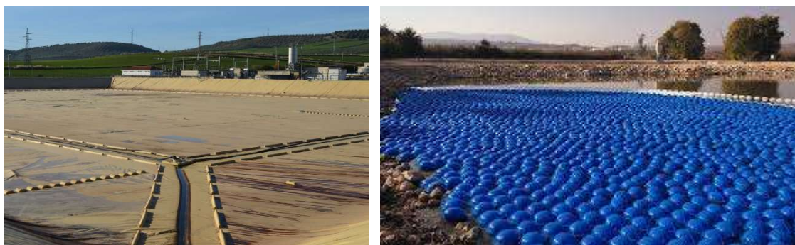
Figure 4-22: Given many existing ponds, mainly for irrigation, covering them is essential to avoid evaporation losses, using continuous floating covers (left image) and discontinuous ones, such as floating balls (right image). These systems offer additional advantages: they prevent algae proliferation, extend the pond's useful life, and reduce water salinity.
