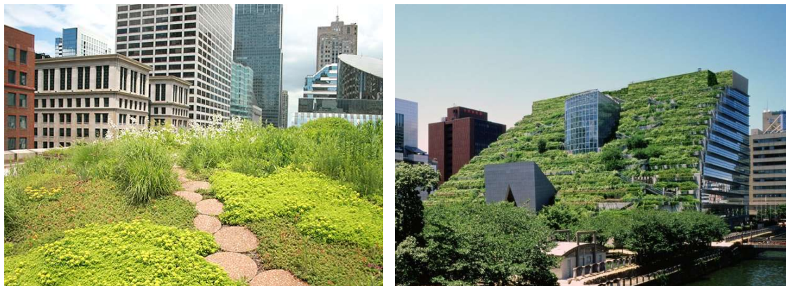
Figure 4-14: The installation of vegetation on rooftops generates many co-benefits. In addition to reducing and slowing stormwater runoff in urban environments, they produce oxygen, provide shade, and reduce heat in cities (in the image on the left the Chicago City Hall, USA, and on the right ACROS-Fukuoka Prefectural International Hall, Japan).
