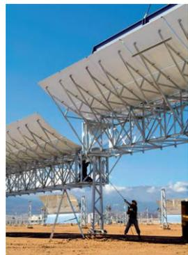
Fig. 21: Parabolic trough [12]
