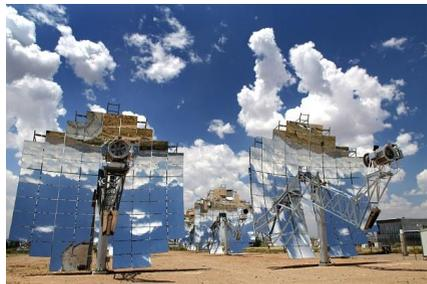
Fig. 23: Dish system with stirling motor [13]
