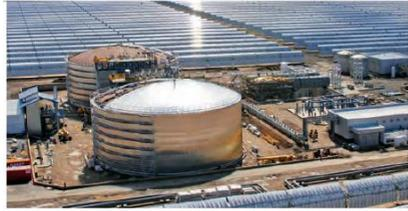
Fig. 73/74: CSP-plants with mirror (left) and trough (right) system and integrated storage tanks using molten salt [32], [33]
