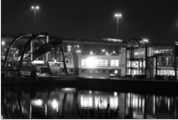
Photo 10. Platform during night.
