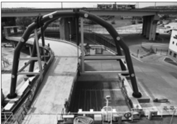
Photo 9. Movable platform with A1 motorway at back.
