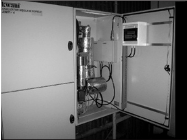
Fig. 9. AWP4 carbon-in-ash monitor installed on an OP-230 boiler
