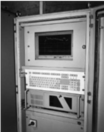
Fig. 3. Control / data processing cabinet of the APF system
