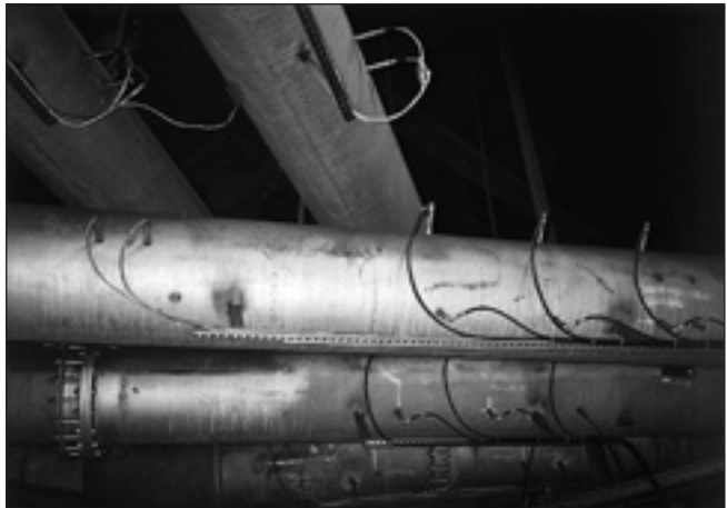
Fig. 4. Measuring probes of the APF system installed on a PF duct of an OP650 boiler
