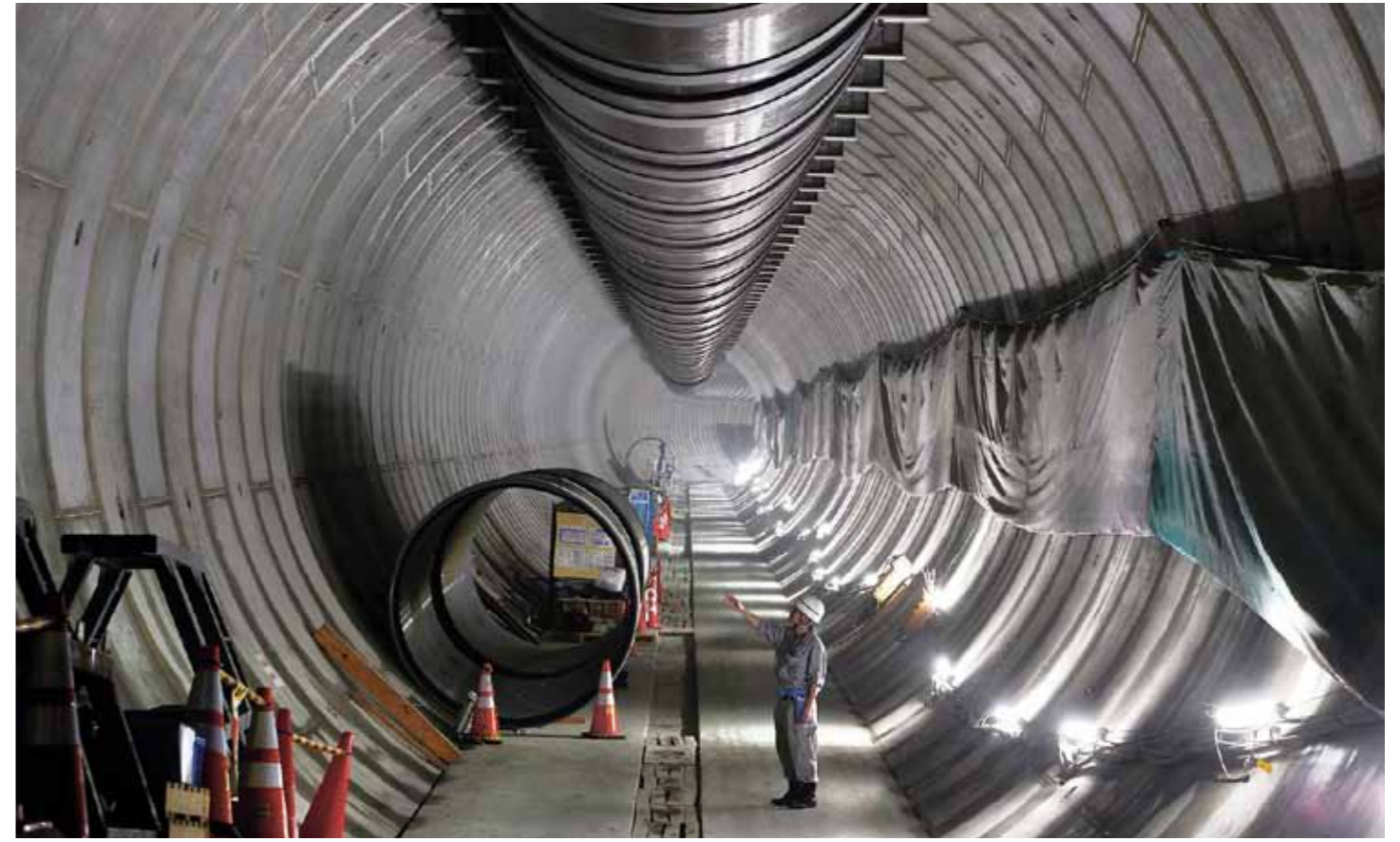
A worker points to the wall of a section of the Furukawa reservoir project being built in central Tokyo on Aug. 7. When completed in 2016, the 3.3-km-long subterranean reservoir will be able to hold 135,000 cu. meters of water, enough to fill 54 Olympic-sized swimming pools. BLOOMBERG
