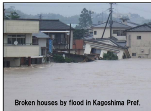
Broken houses by flood in Kagoshima Pref.
