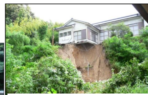
Landslide under the houses in Kagoshima Pref.
