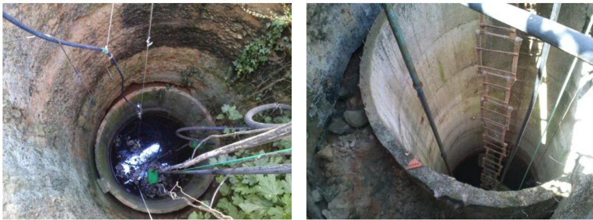
Figure 51 – Traditional large diameter wells potentially suited for injection of harvested water
