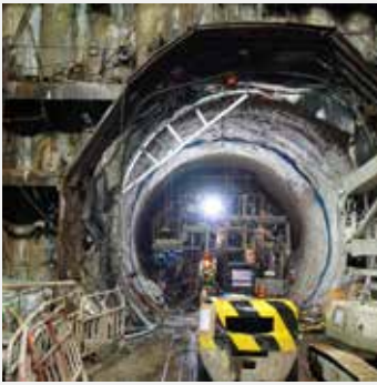
Engineering infrastructure, such as this underground metro tunnel, is essential for sustainable development. © Mr Pung Chun Nok, Hong Kong Institution of Engineers
